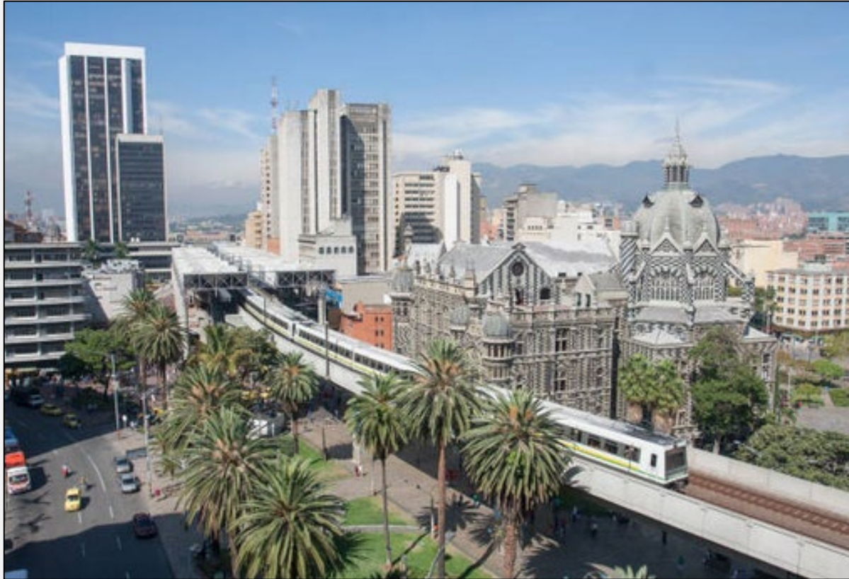
An above ground new rail system moves people within the city and transit stations are clean and offer something to look at (the New York City subway system it isn't!)
